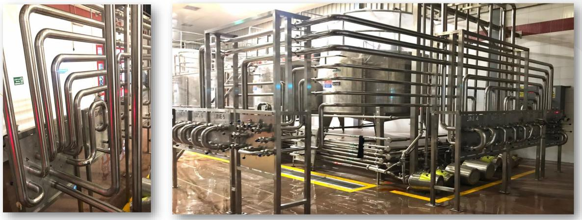
Pipeline design and installations for CIP unit from ADUE in Coca Assiut
